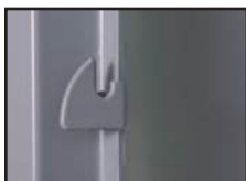
Main door latch hooks welded to frame
